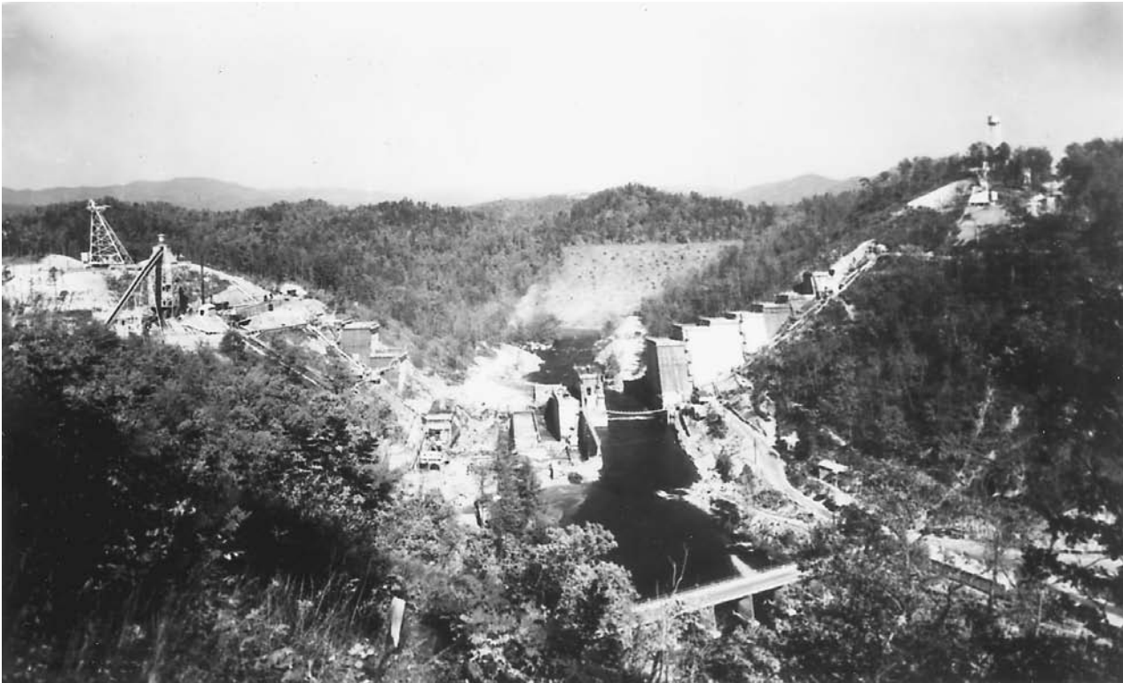
The Hiawasse Dam in North Carolina, under construction by the TVA in the late 1930s. FRANKLIN DELANO ROOSEVELT LIBRARY
