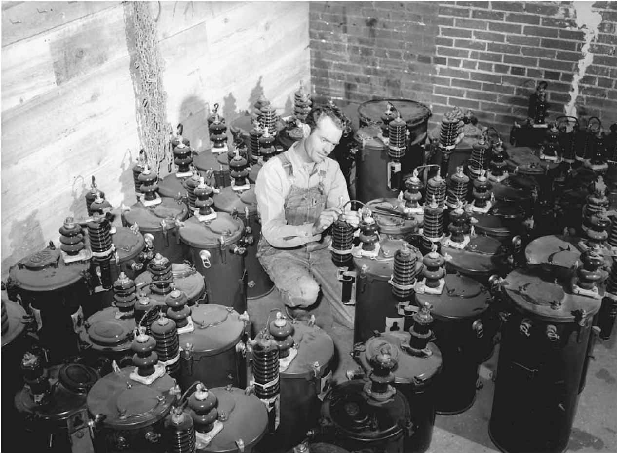
An REA employee checks transformers at the REA cooperative headquarters in Hayti, Missouri, in 1942. LIBRARY OF CONGRESS, PRINTS & PHOTOGRAPHS DIVISION, FSA/OWI COLLECTION
