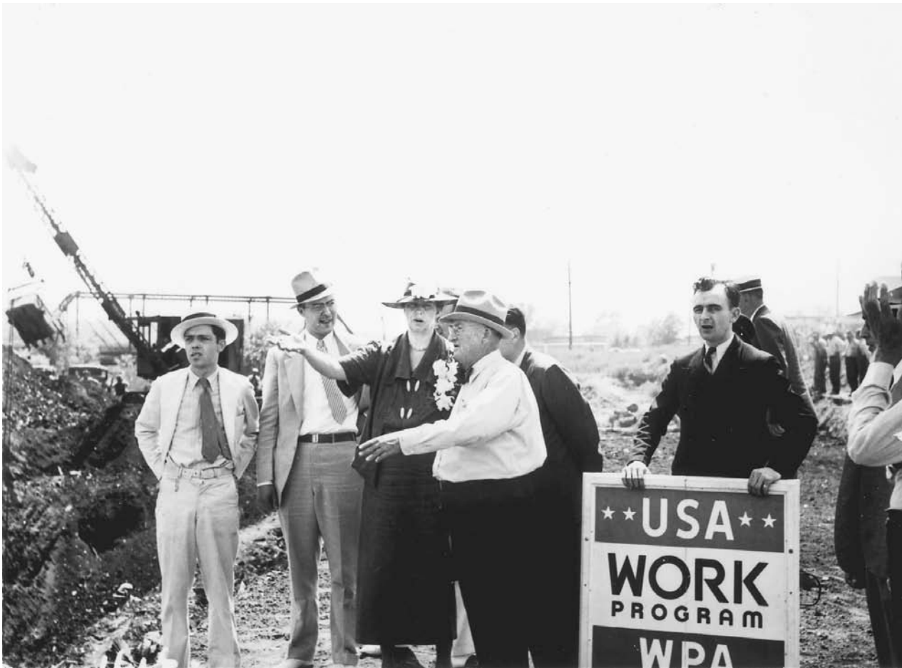
Eleanor Roosevelt visits a WPA construction site in Des Moines, Iowa, in June 1936. FRANKLIN DELANO ROOSEVELT LIBRARY
