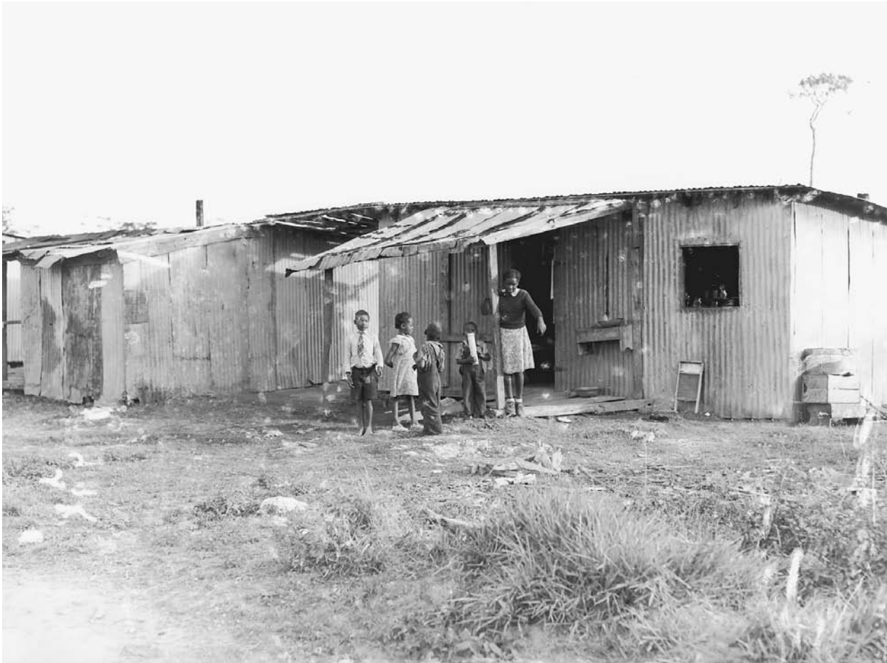
Dilapidated quarters for migrant agricultural laborers in Homestead, Florida, in 1939. LIBRARY OF CONGRESS, PRINTS & PHOTOGRAPHS DIVISION, FSA/OWI COLLECTION
