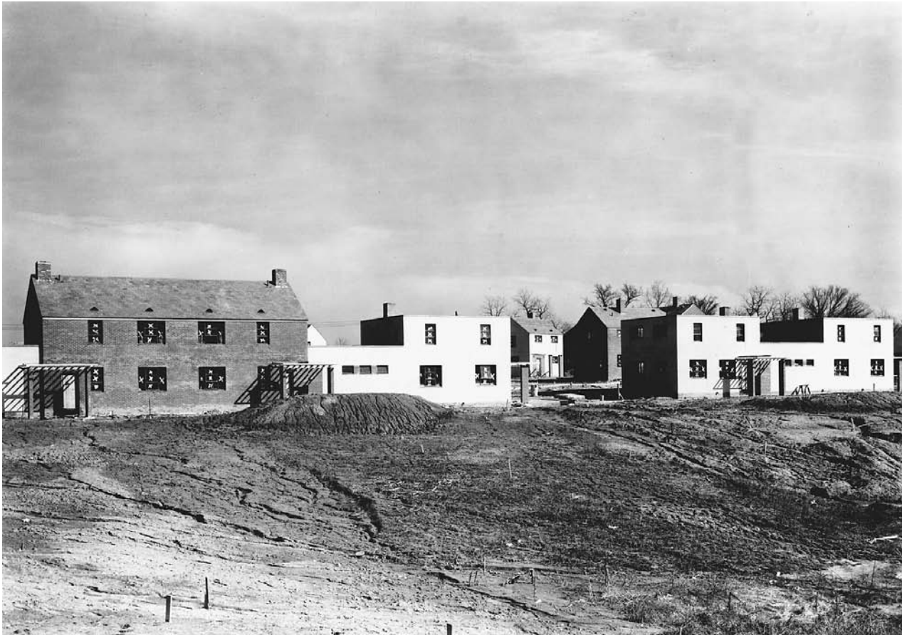
This housing project under construction in Greenhills, Ohio, in 1937 was one of numerous Resettlement Administration initiatives.
