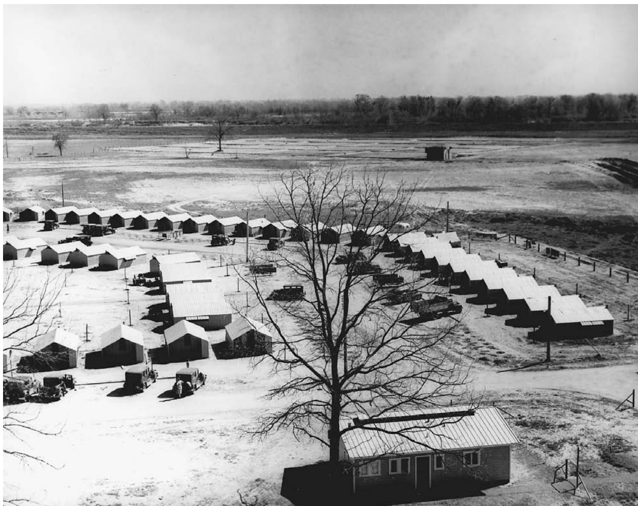
This newly constructed Farm Security Administration camp for seasonal workers, photographed in 1940 near Yuba City, California, boasted steel shelters, rather than the tents found in many older camps. The camp also included a clinic. NATIONAL ARCHIVES AND RECORDS ADMINISTRATION
