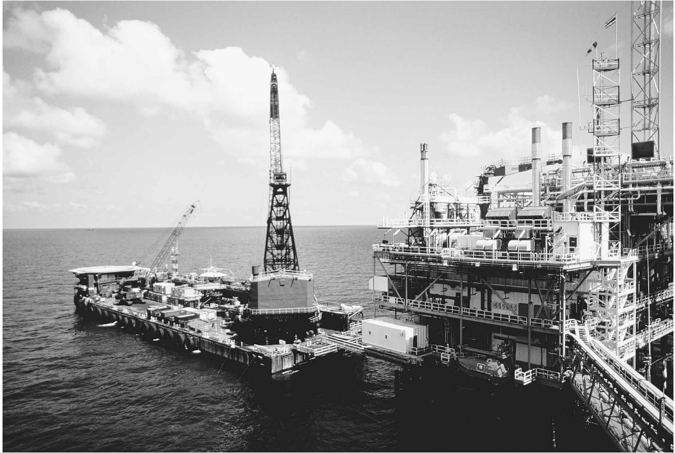
Gas production platform under construction in the Gulf of Thailand. (Corbis-Bettmann)
